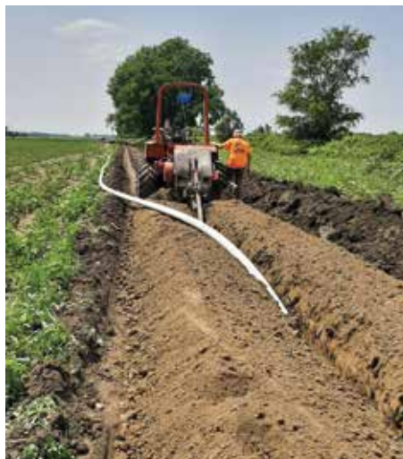
Installing 4" on Timber Road
