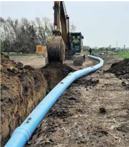
Installing 14" Mainline on 304th Street
