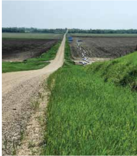
Installing 14" Mainline on 304th Street
