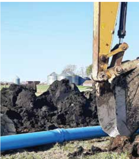
Installing 12" on 458th and 304th
