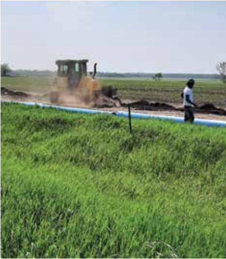
Installing 14" Mainline on 304th Street
